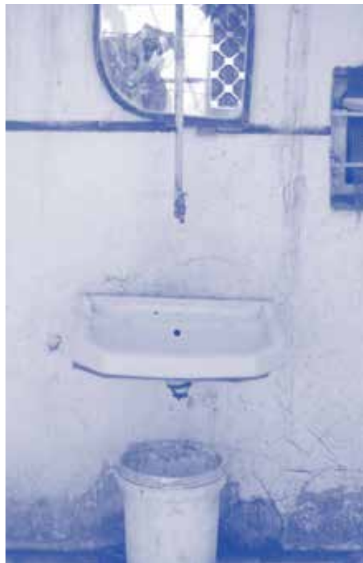
fig. 90: Self-made waste water collection (own photograph)
